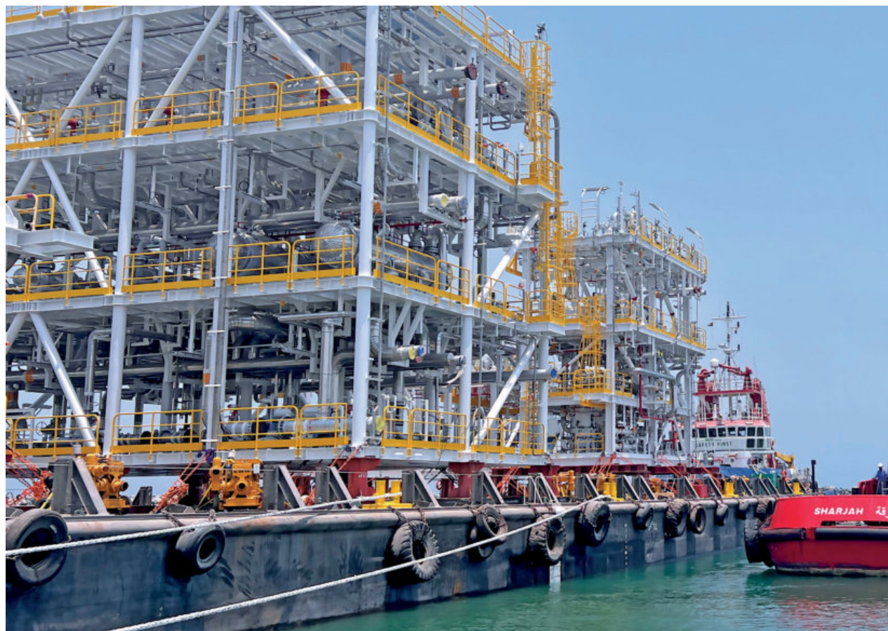
Picture of an Erhardt Projects site with industrial equipment
