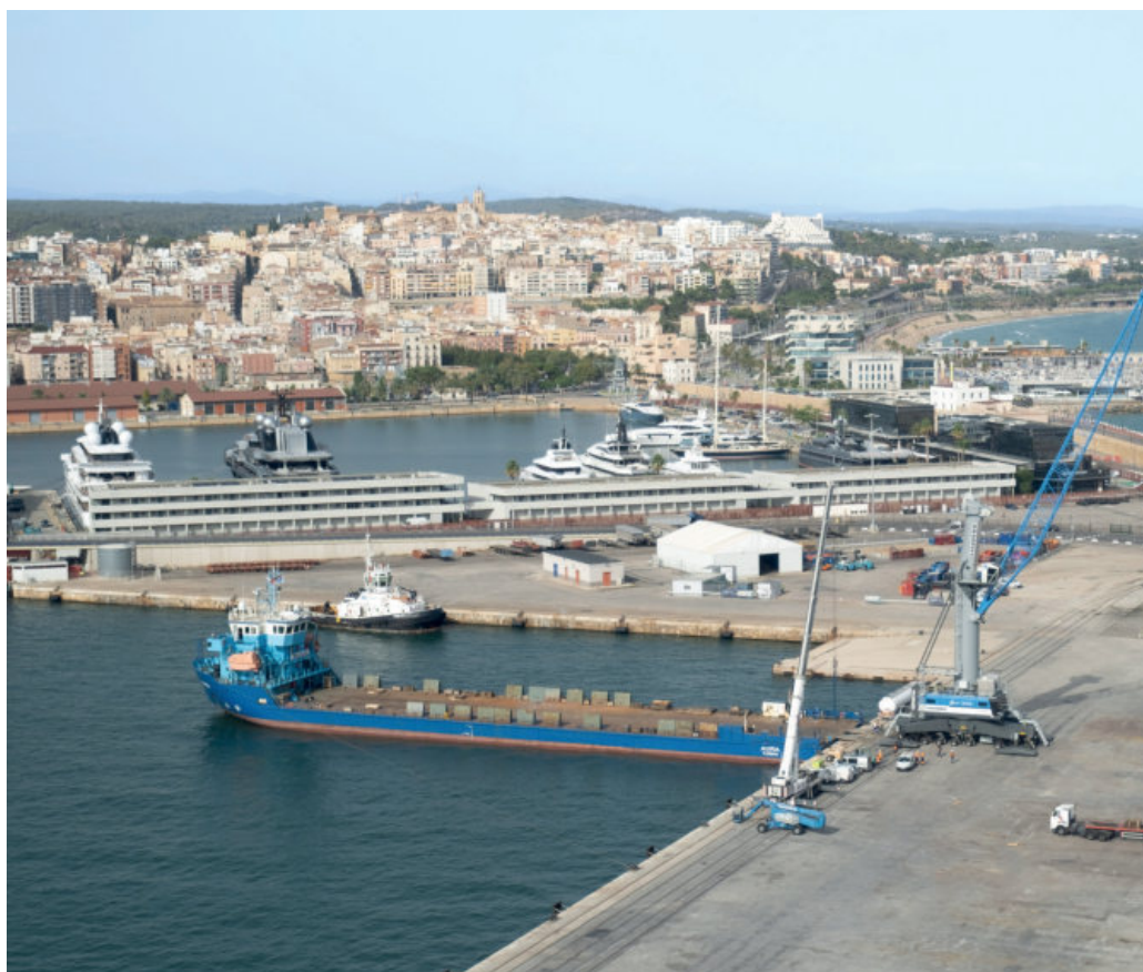
New Ership crane for its terminal in the port of Tarragona.
